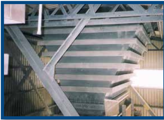
Hopper lined with INERTIA™ Tactical Wear Plate .
