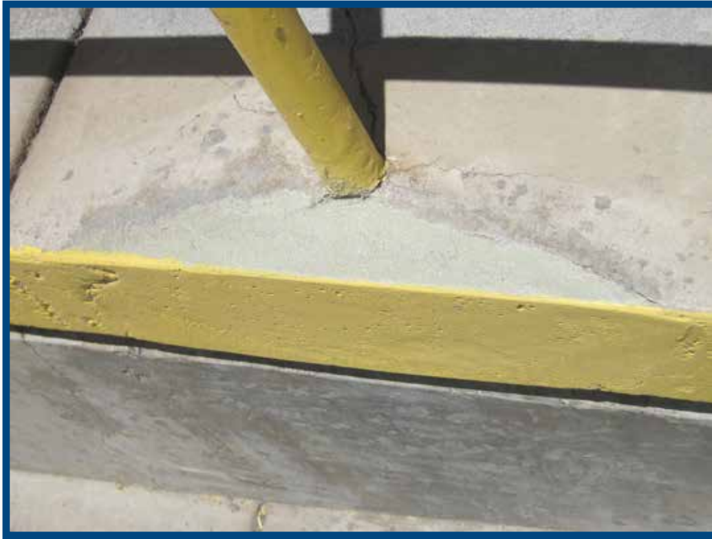
Wear-Concepts' Fortify™ used to patch damaged dock edge.
