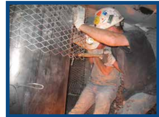
Extruded mesh being installed.
