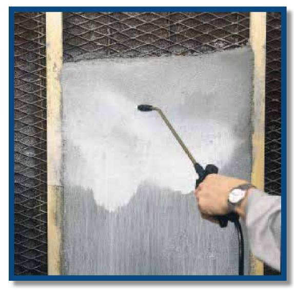
Wear-Con Densit® Curing Compound being applied to sectioned Densit® WearFlexTM.
