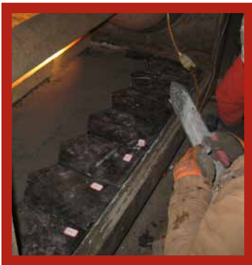
Installing Cast Basalt Tiles.
