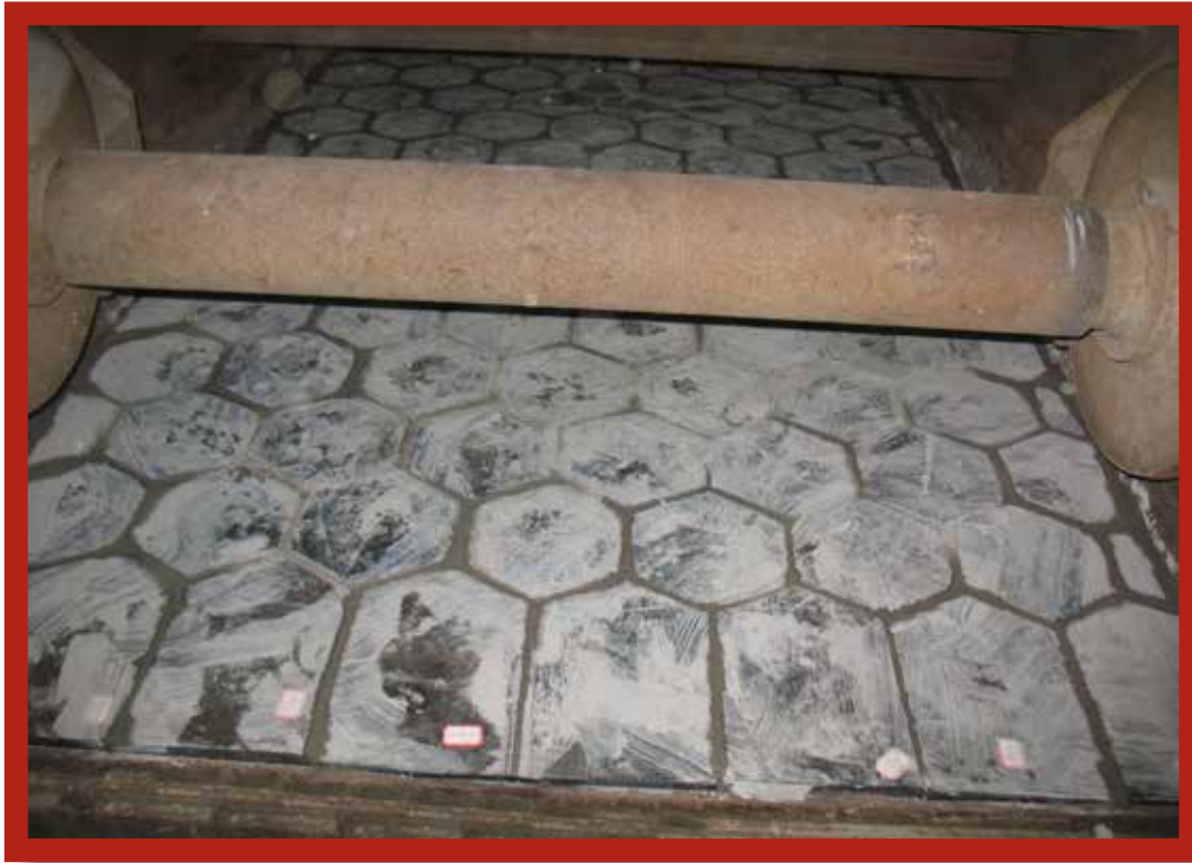
Newly installed Cast Basalt Tiles in a drag conveyor.
