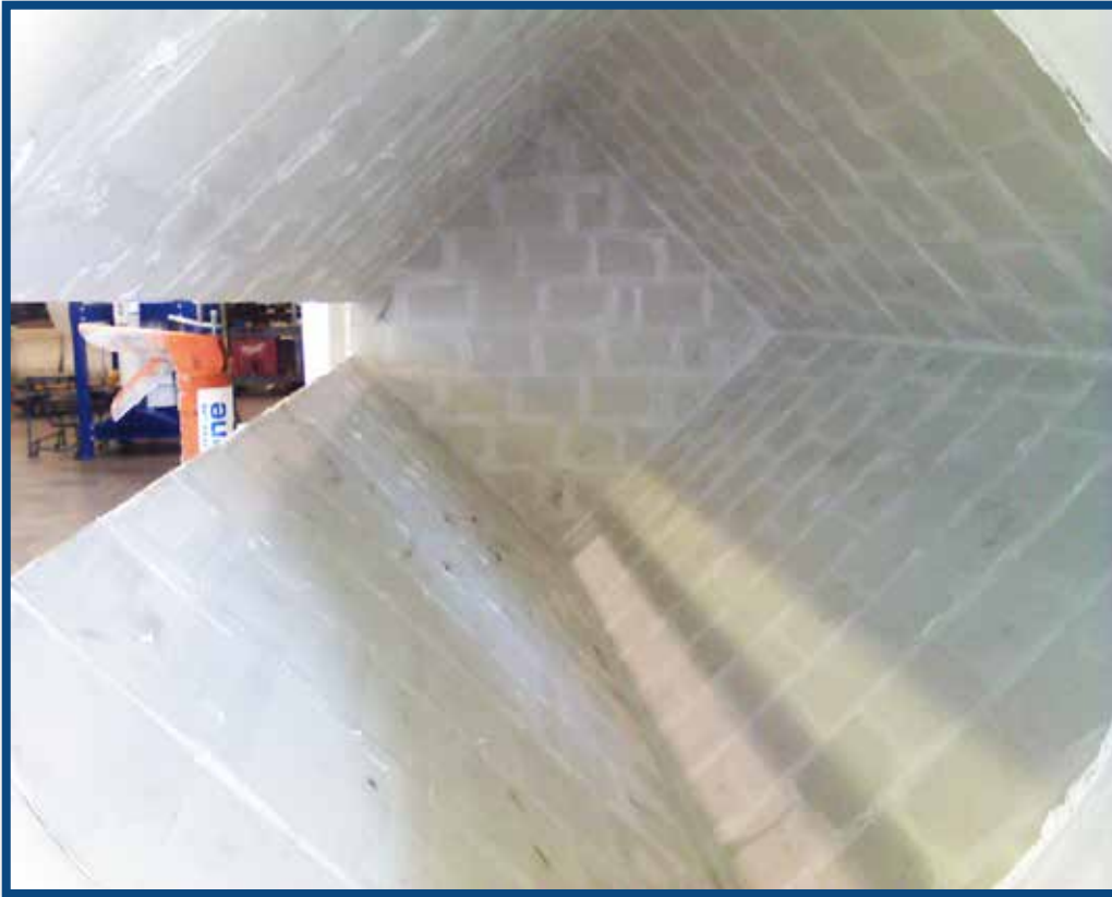
WC90™ Plain Tile installed.
