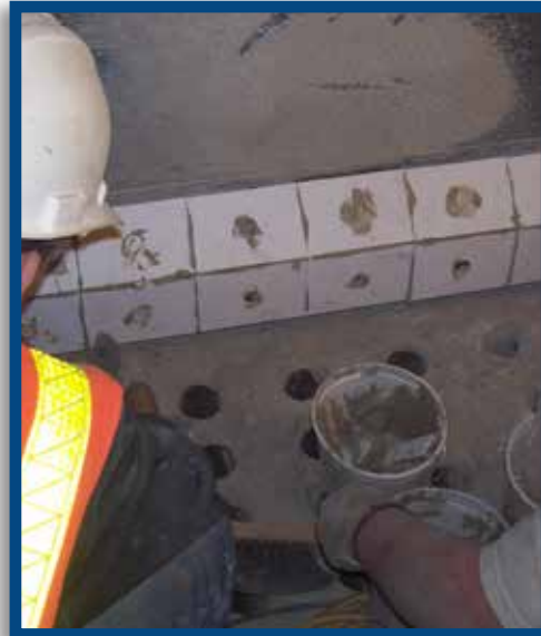
WC90™ Plain Ceramic HexTile & Weldable Ceramic Tile installed with Cerami-Bond™ .
