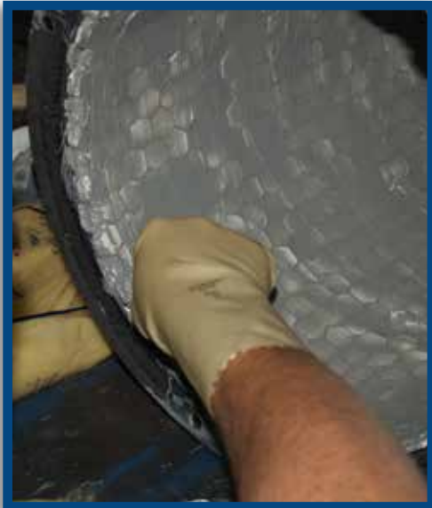
WC90™ Plain Ceramic HexTile & Weldable Ceramic Tile installed with Cerami-Bond™ .
